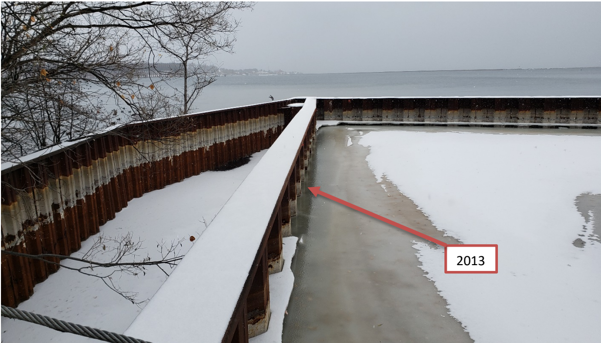
Photo No. 3 – North Sheet Pile Wall
