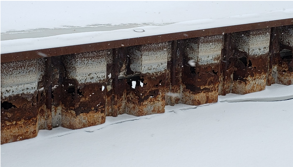
Photo No. 8 – Interior Wall Condition
