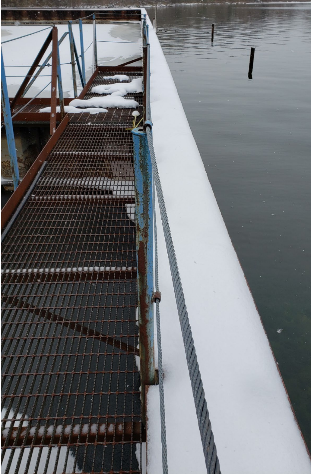
Photo No. 7 – East Wall Alignment
