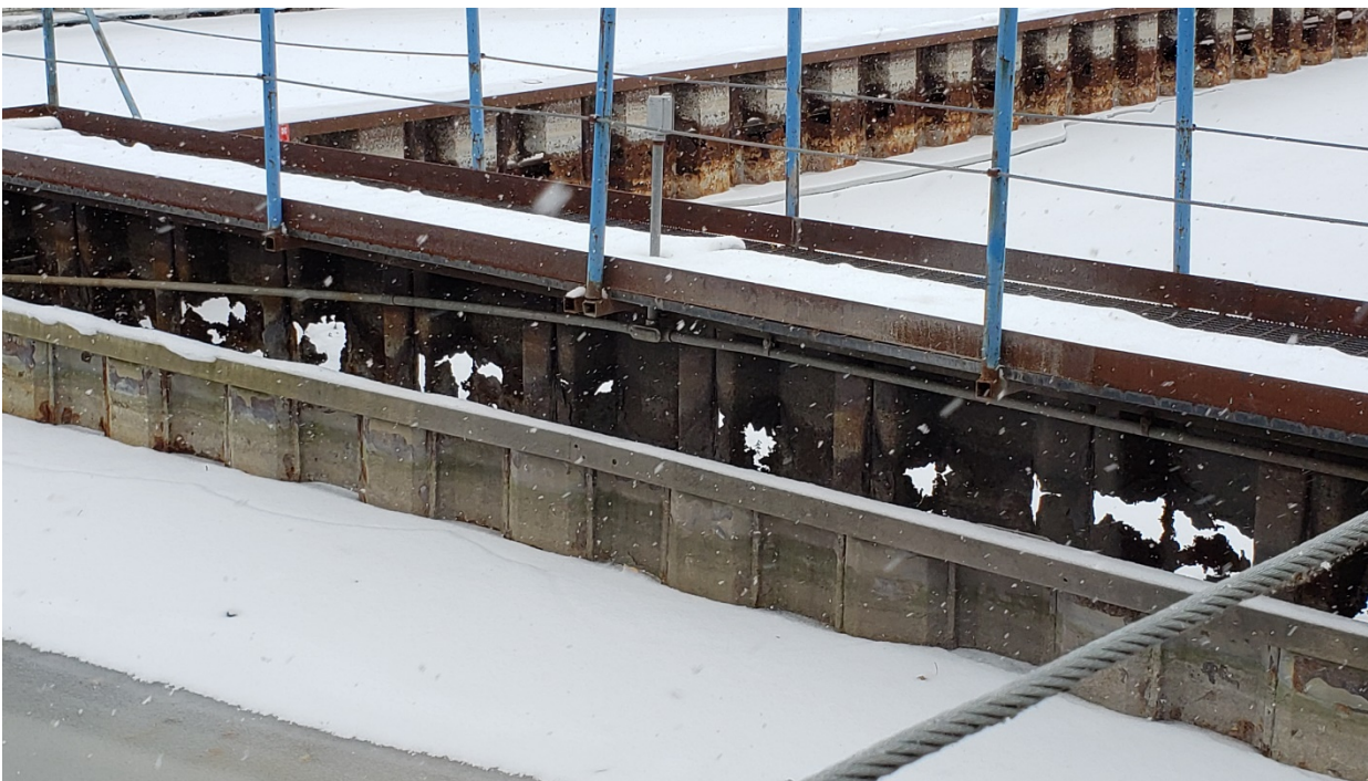
Photo No. 9 – Adjacent Interior Walls
