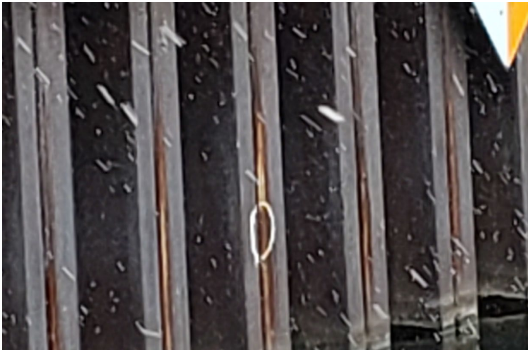
Photo No. 6 – East Wall Joint to Monitor
