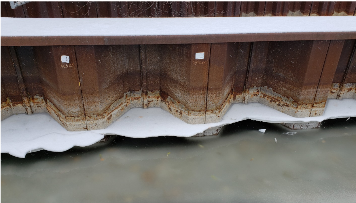
Photo No. 4 – North Sheet Pile Wall Condition
